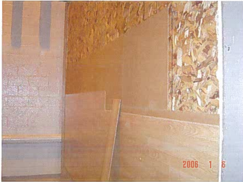
Installation of Sub Floor and Laminate
